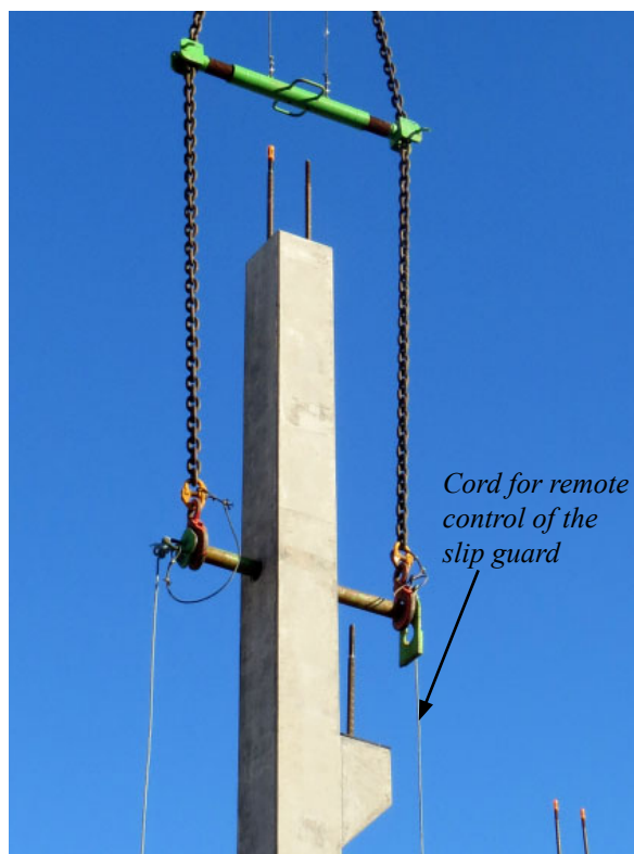
Figure 16. Whole system assembled, including cords for removing the slip guard and mounting shaft.
