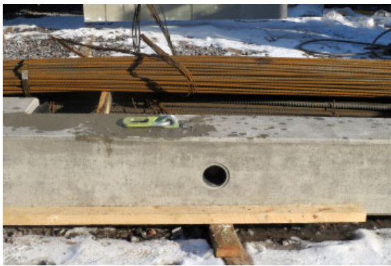
Figure 7. Hole for mounting shaft in precast element.
