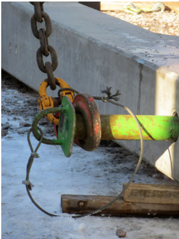
Figure 13. Attaching the mounting shaft to the lifting sling with steel wire.
