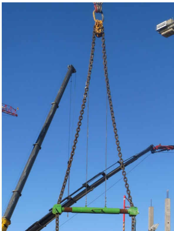
Figure 15. Attaching the rope strut to the oblong ring with steel wire.
