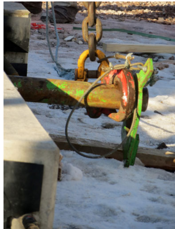
Figure 14. Attaching the slip guard to the lifting sling with steel wire.
