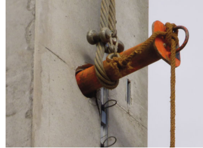
Figure 24. Slings attached with rope loop and shackle.
