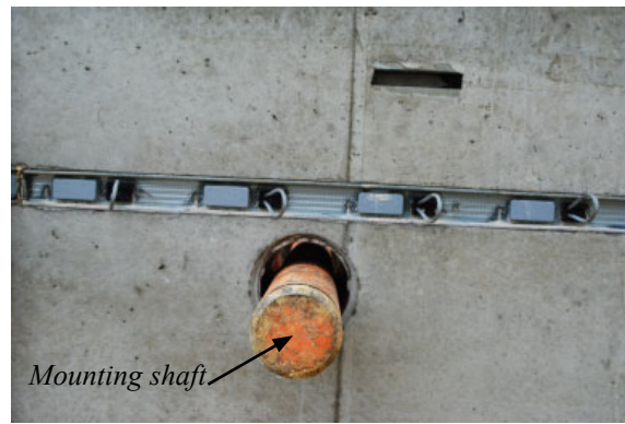
Figure 8. Mounting shaft placed in the hole.
