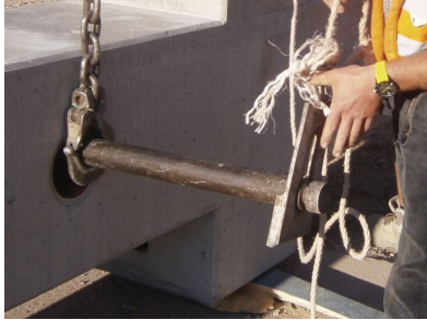
Figure 22. Slings attached with hooks.
