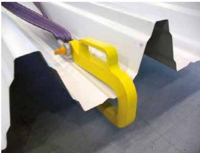
Figure 8. Placing the hook on the load.
